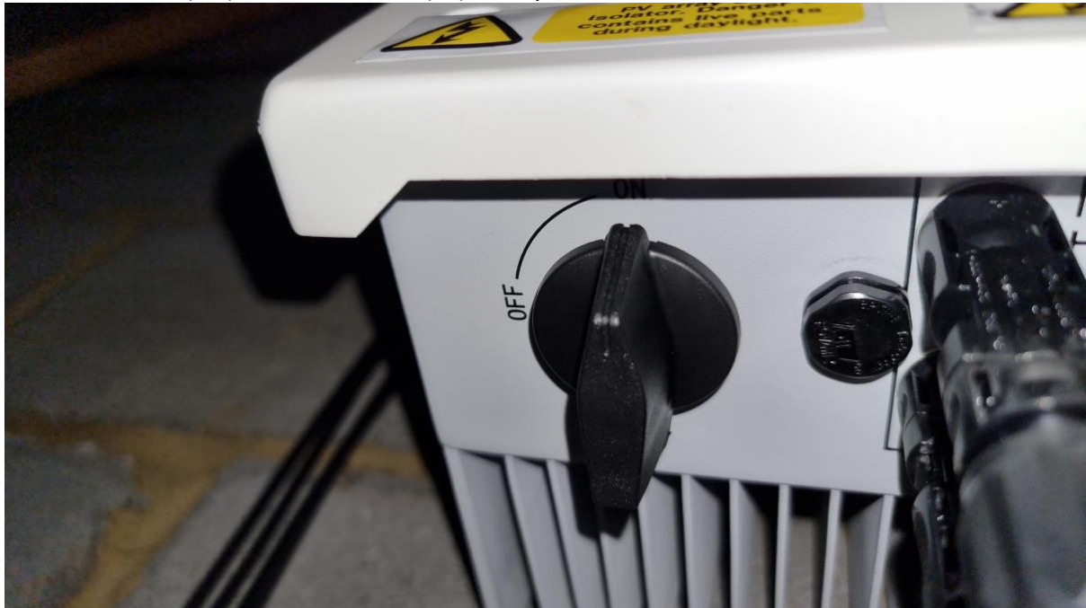
Fig 28. Turn on the PV isolator switch.
