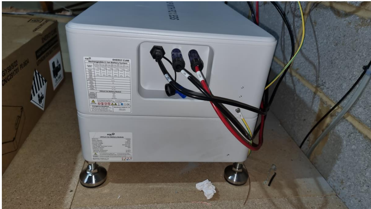
Fig 2. Existing connections before the upgrade is done. (Battery terminals, CAN network cable and Earth cable)
