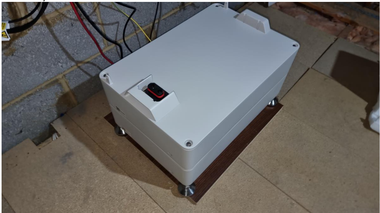
Fig 21. New slave module added to the existing stack of slave(s).
