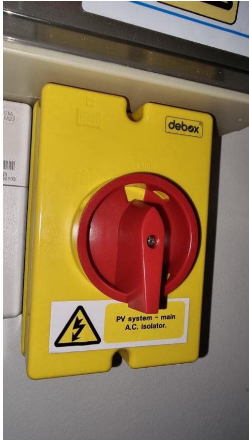
Fig 30. AC Isolator switch near the consumer unit to 'On' position.
