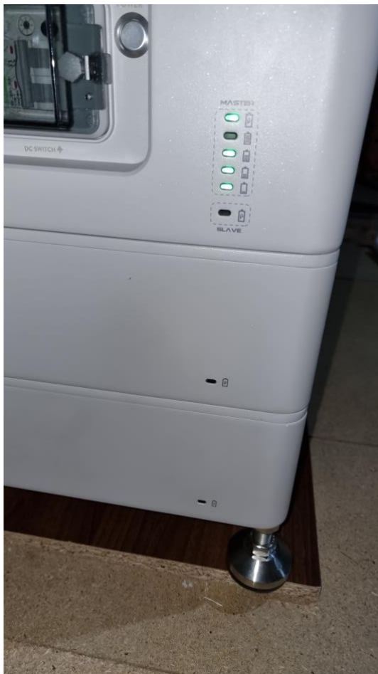
Fig 37. The battery module displaying 3 of the four LEDs flashing confirming the status of charge on the battery.
