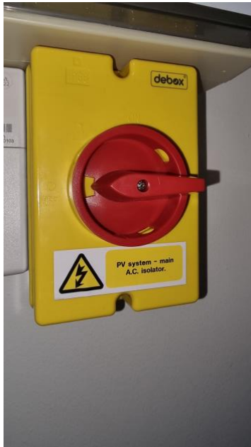
Fig 14. Isolator switch next to consumer unit to 'Off' position.
