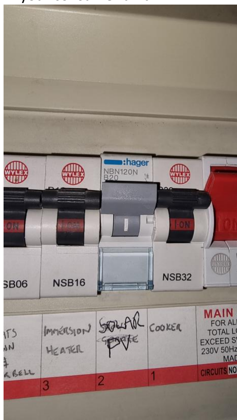
Fig 29. Breaker switch in consumer unit to 'On' position.
