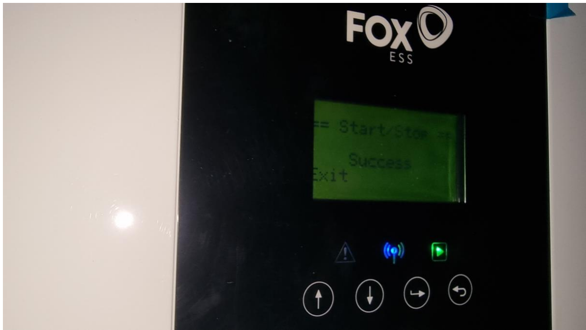
Fig 34. Screen showing successful start operation on the inverter.
