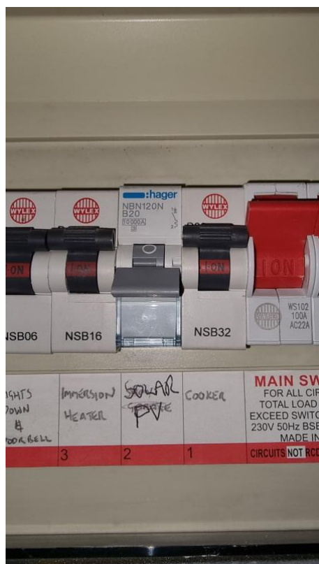
Fig 13. Breaker switch to 'Off' position.
