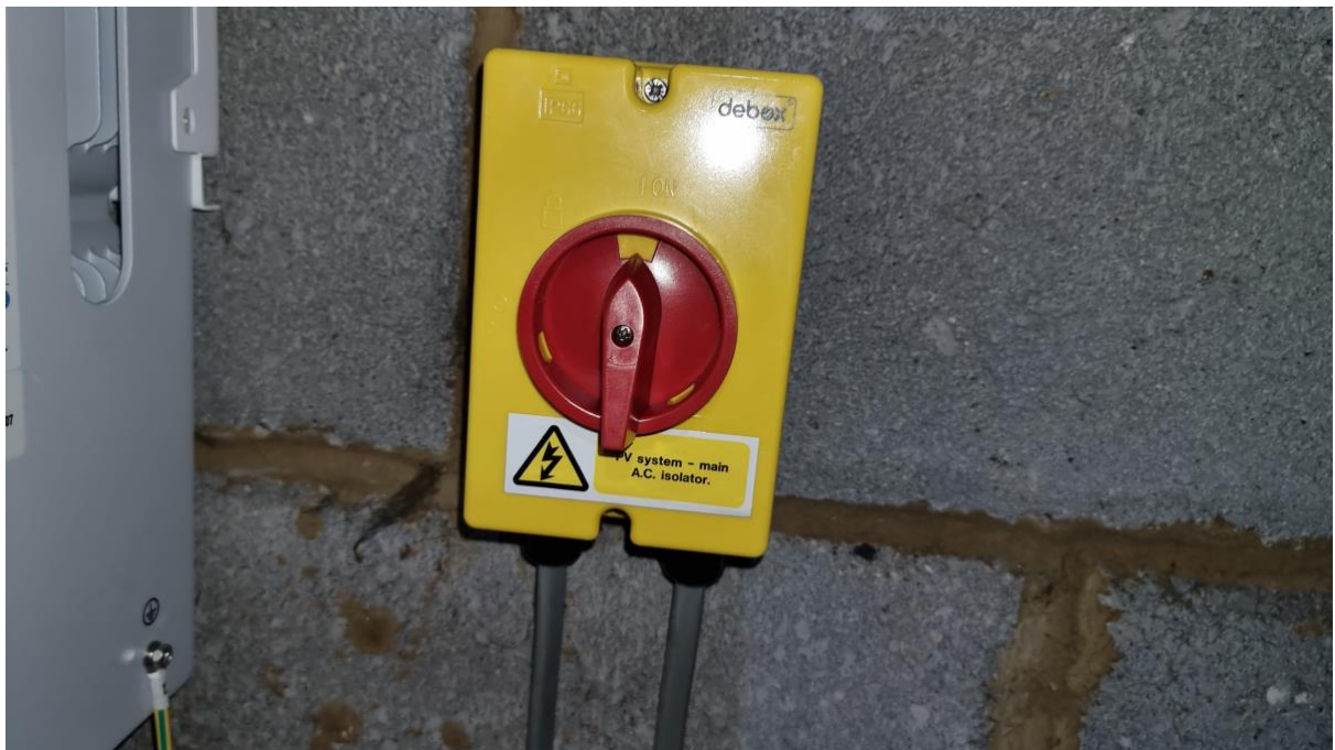
Fig 31. AC Isolator switch near the inverter unit to 'On' position.
