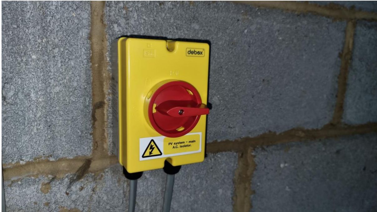
Fig 12. AC isolator switch next to the inverter to 'Off' position.
