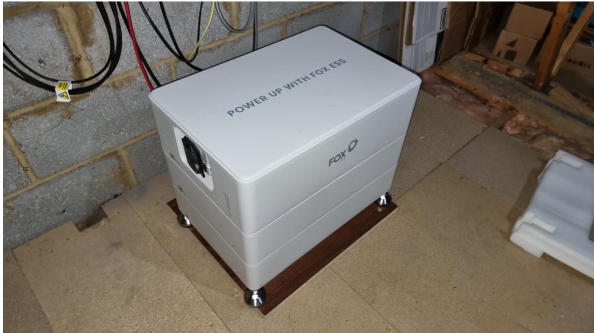
Fig 22. All battery modules in place.
