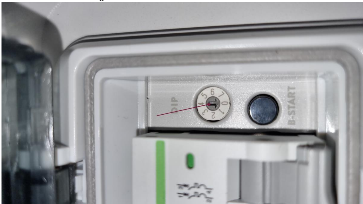
Fig 25. Dip switch position highlighted with red arrow before upgrade.
