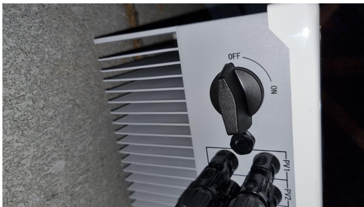
Fig 11. PV isolator switch to 'Off'
