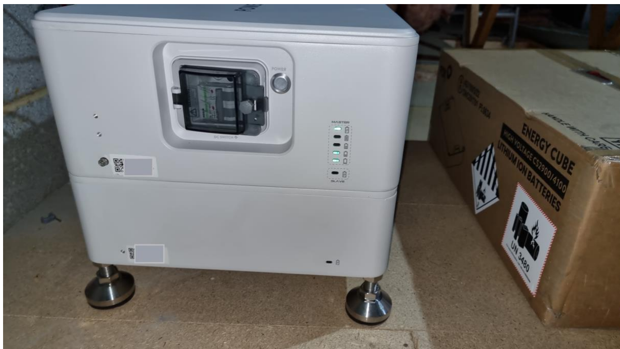
Fig 3. Existing module setup before the upgrade is done. (Battery Master and Slave module(S))
